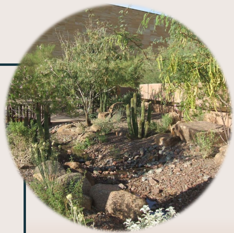
Example of a GSI: Bioswale
